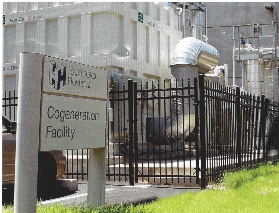
FuelCell Energy's 1.4-MW MCFC power plant at Hartford Hospital in Connecticut. (Source: FuelCell Energy Inc.)
