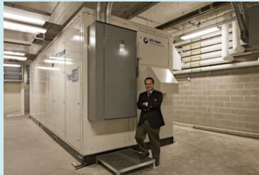
Bottom: 360 State Street, New Haven, CT
