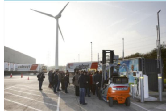
Fuel cell forklift fueling at Colruyt's renewable hydrogen station
