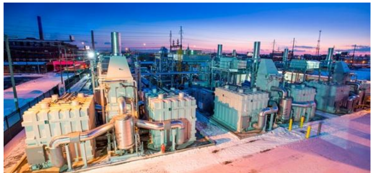
14.9-MW Dominion Bridgeport fuel cell in Bridgeport, Connecticut, operated and maintained by FuelCell Energy.
