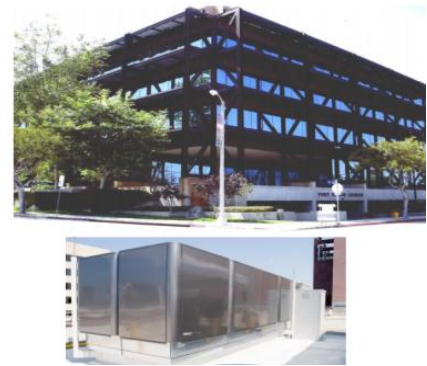
A fuel cell at the Port of Los Angeles powers the Administration building.
