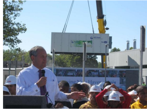
Fuel cell installation at Roberto Clemente Leadership Academy and Hill Central School (New Haven, Connecticut)
