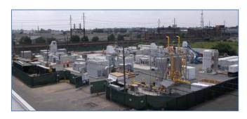
In May 2013, energy company **Dominion**, broke ground on a 14.9-MW fuel cell power – generating facility in Bridgeport, Connecticut – enough electricity to power approximately 15,000 homes. FuelCell Energy will build, operate, and maintain the facility, which will include five Direct FuelCell® stationary fuel cell systems and an organic rankine turbine that will
