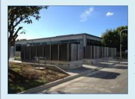
**Honda** installed five Bloom Energy fuel cell systems (totaling 1 MW) to provide 25 percent of the electricity needs for its 1.13 million square feet (sq. ft.) of office space, research, design and development operations, and parts distribution center in Torrance, California. The fuel cells, which run on natural gas, will reduce Honda's carbon dioxide emissions by approximately 16 million pounds over 10 years.
