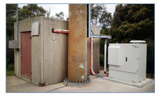
Queenstown, Tasmania. A lightning strike to the mobile base station's AC rectifier meant the AC power couldn't be converted to DC power to run our equipment.... So the back-up power supply had automatically kicked in to keep the base station running.
