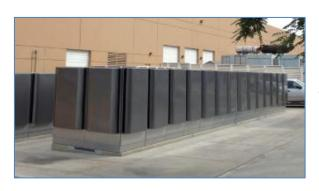
In 2012, Life Technologies installed a 1-MW Bloom Energy fuel cell system at its Carlsbad, California, campus. The fuel cells were installed in an uninterruptible power configuration to protect Life Technologies' labs, freezers, and critical experiments and provide 60 percent of the electricity needs for the facility while reducing carbon emissions by 30 percent. The company previously installed a 1-MW fuel cell system at its Pleasanton, California facility.
